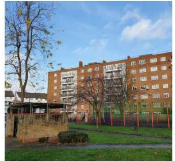
3 View of refuse store on site towards North West
