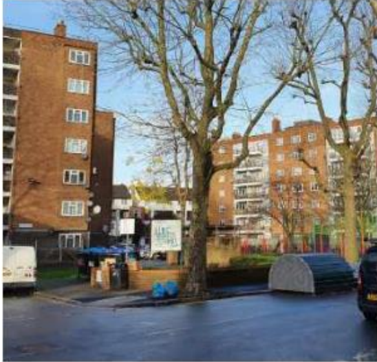
1 View of Longfield Estate towards North West
